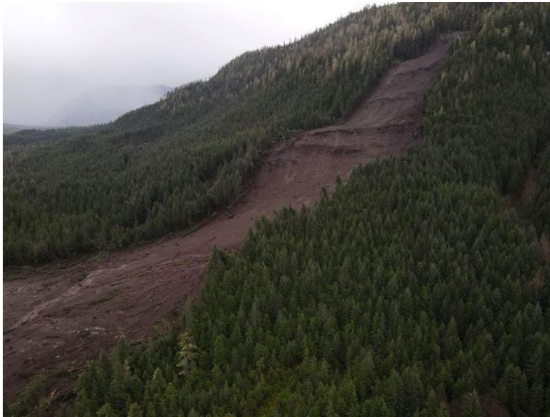
Upslope View of Zimovia Highway Landslide
